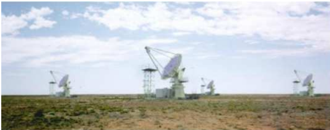
Fig. 6.2. Photograph of the four Cangaroo III Cherenkov telescopes in the Australian outback. The telescopes were arranged in a diamond pattern. Each telescope had a nearby access tower for servicing the camera. The mirrors had a diameter of 10 m.
